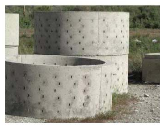
Figure E.4. Dry Well #1 – Structural Prefabricated Chamber.
