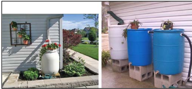
Figure E.1. Rain Barrels.
