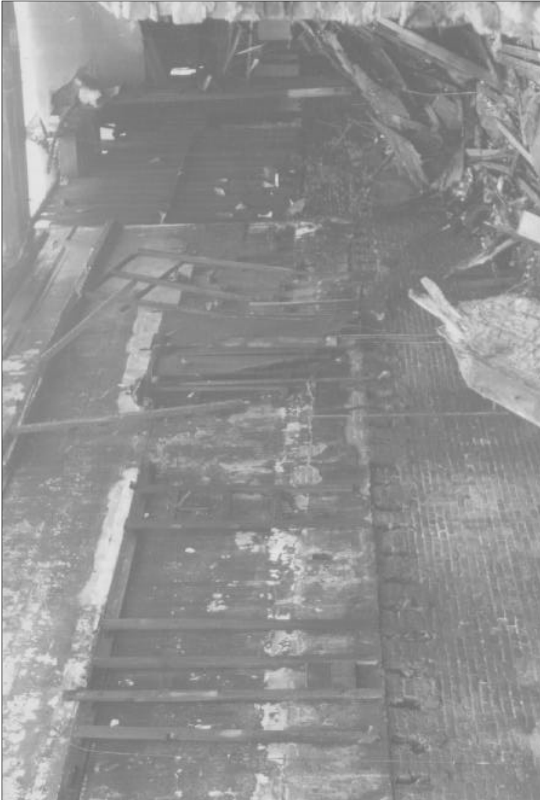
The wall of the front portion of the stationary store remains standing, although the interior is destroyed and the roof has collapsed.
