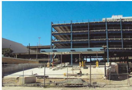
Wilkes-Barre Intermodal Center Nearing Completion.
