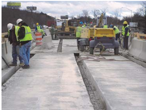
One of Several Bridge Deck Replacement Projects on I-81
