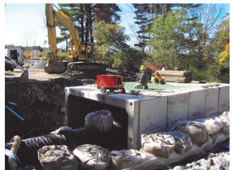
New Box Culvert Over Ackerly Creek on SR 407
